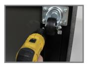
Hold the caster rail set in place as you fasten the screws into the unit through the designated holes.
